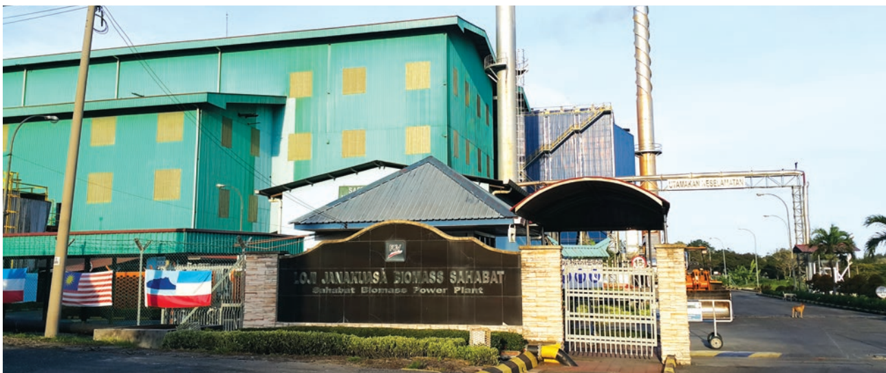
Biomass Power Plant in Sabah
