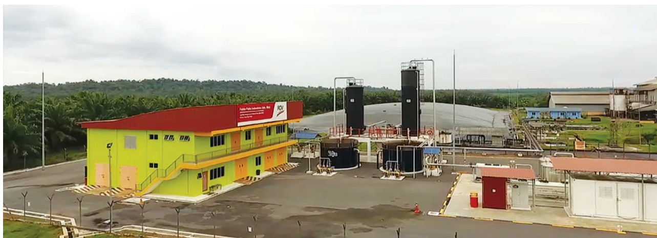
Bio-CNG Plant at Sg. Tenggi Palm Oil Mill
