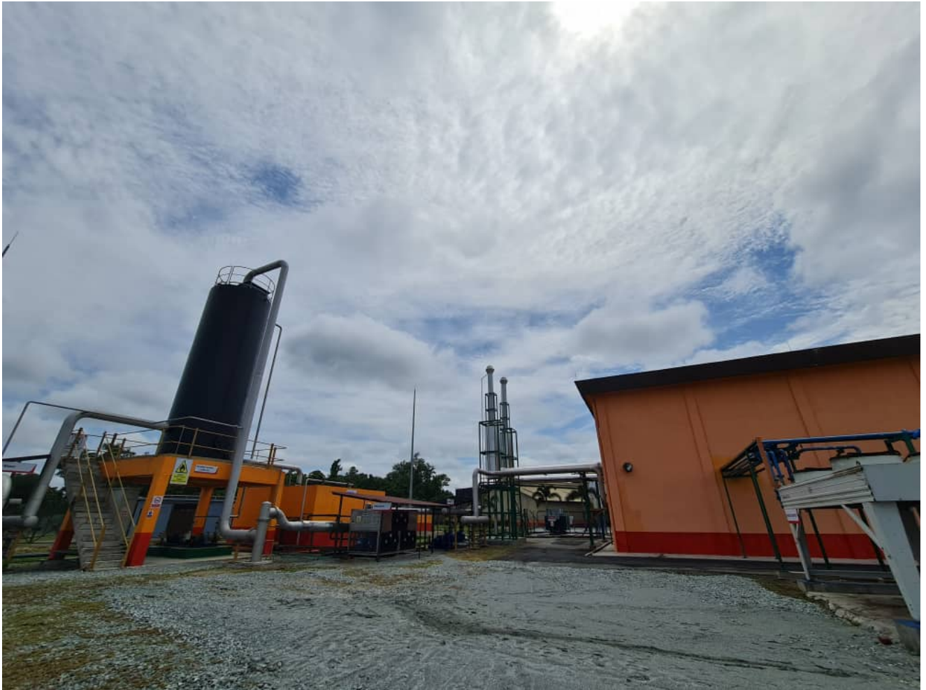
FGV's Triang biogas power plant building
