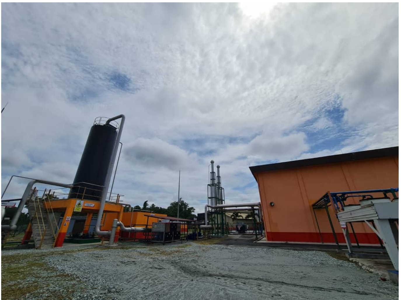
FGV's Triang biogas power plant building
