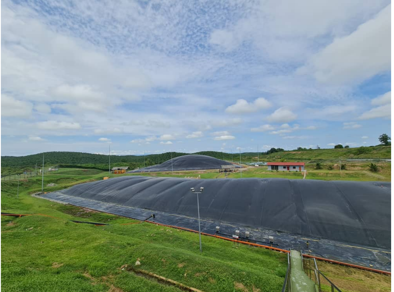
FGV's Triang biogas power plant
