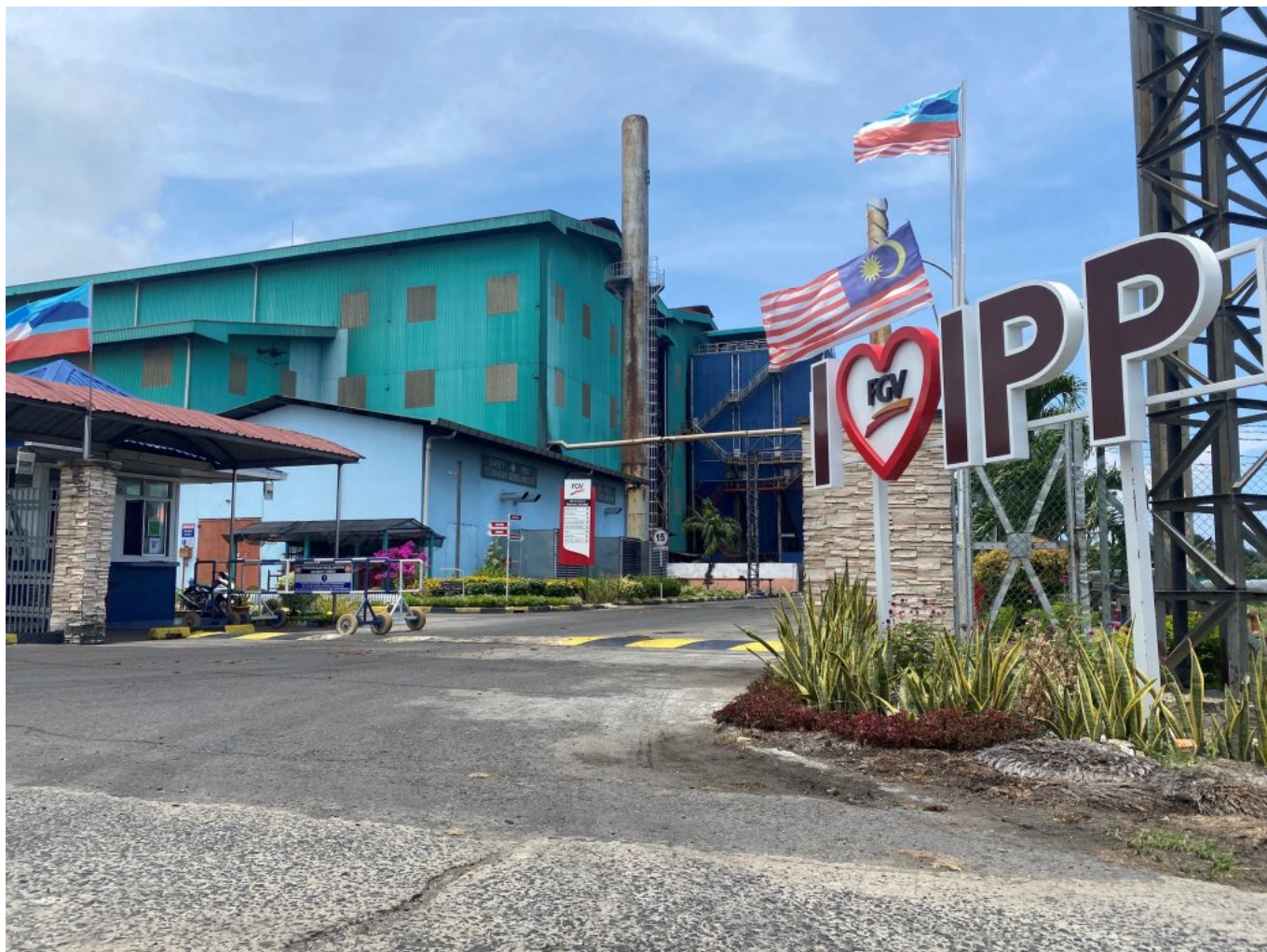
FGV's Sahabat Biomass Cogeneration Plant in Lahad Datu, Sabah
