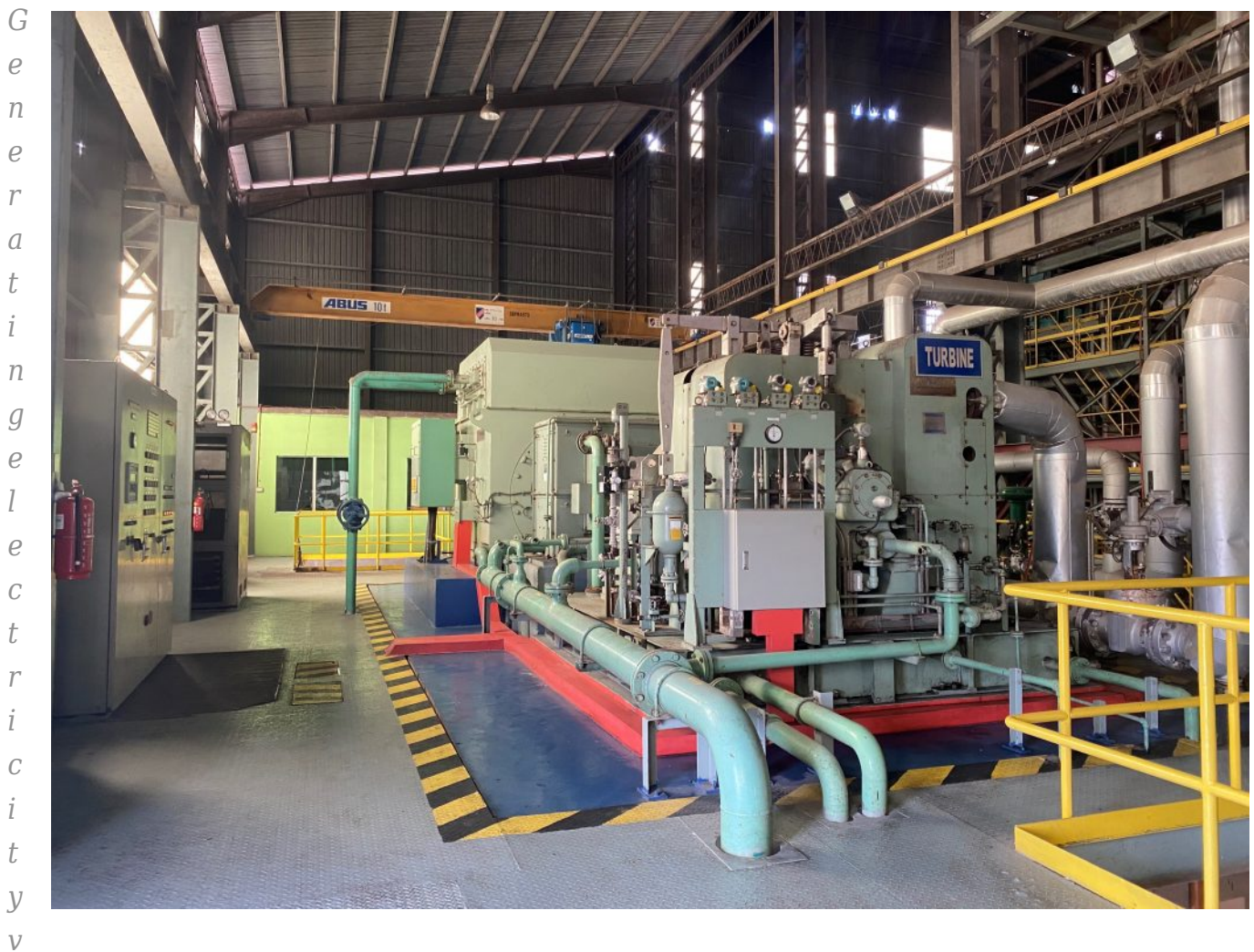
ia steam turbine with a capacity up to 7.2MW
