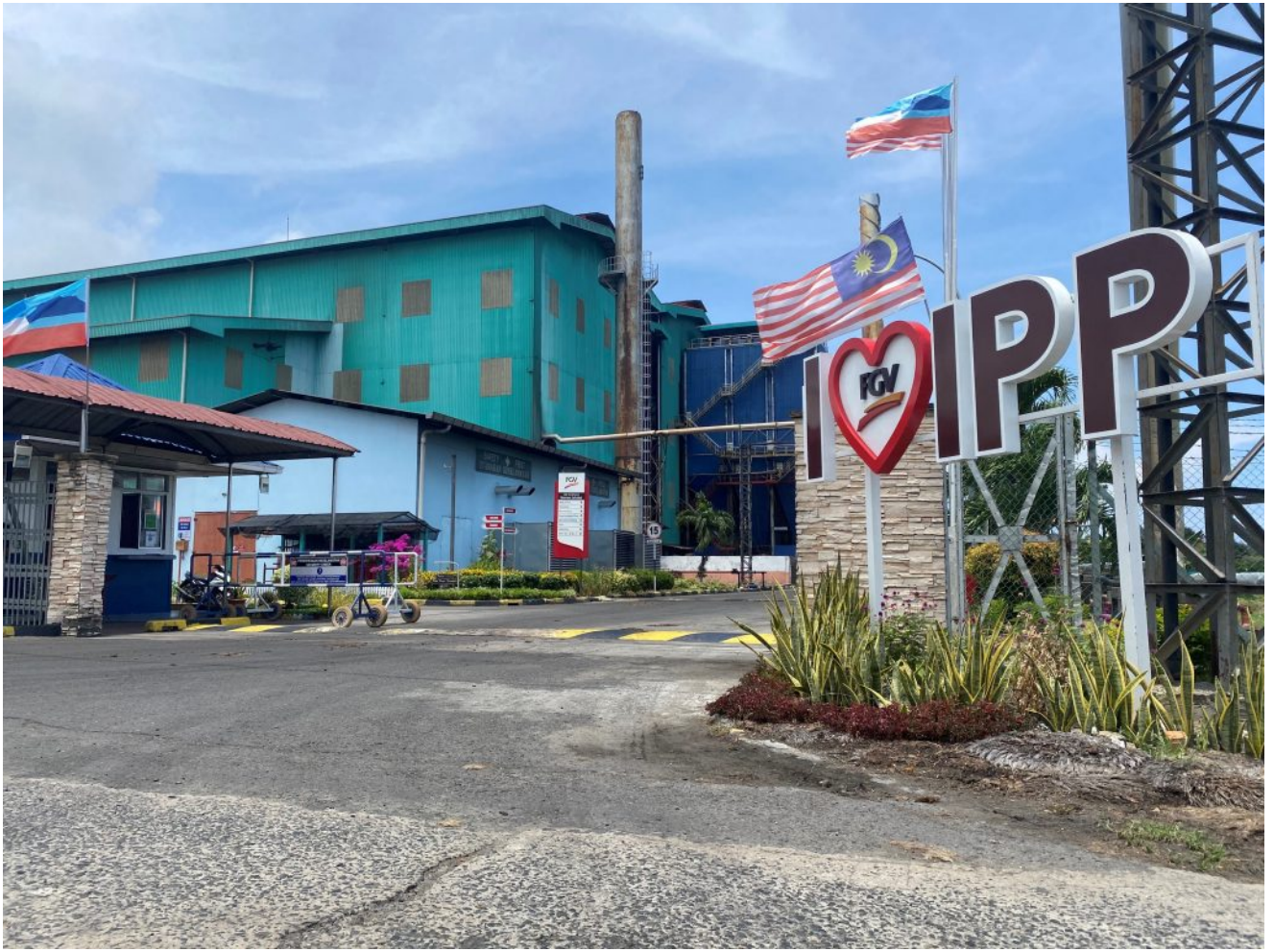
eneration Plant in Lahad Datu, Sabah
